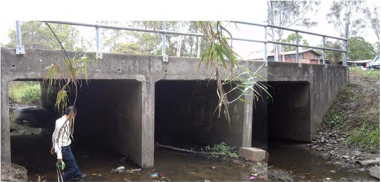
Photo 1 – 3 x 2.8W x 2.05H RCBC under Townson Road looking upstream
