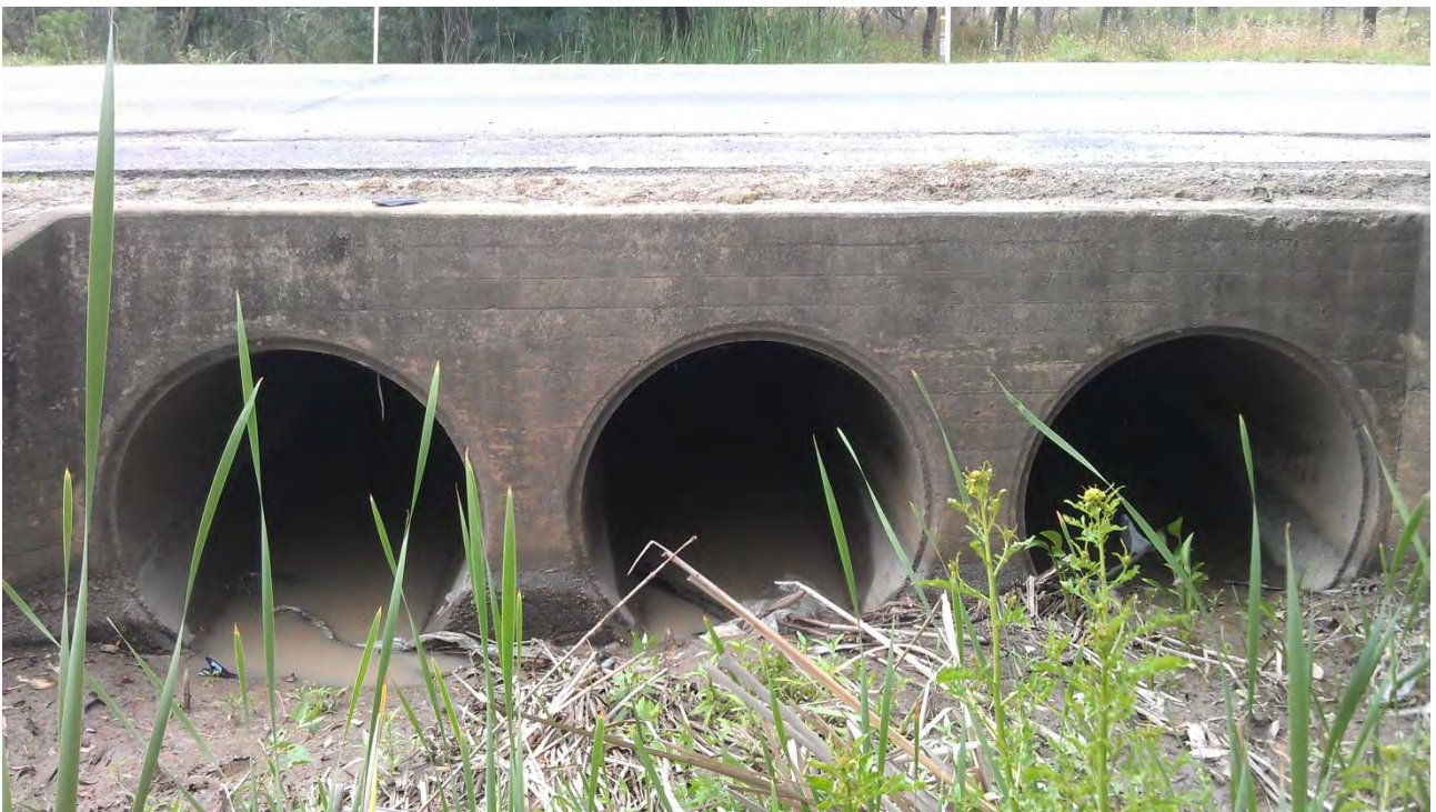
Photo 2 – 3 x 1.05 RCPs under Richmond Road looking downstream
